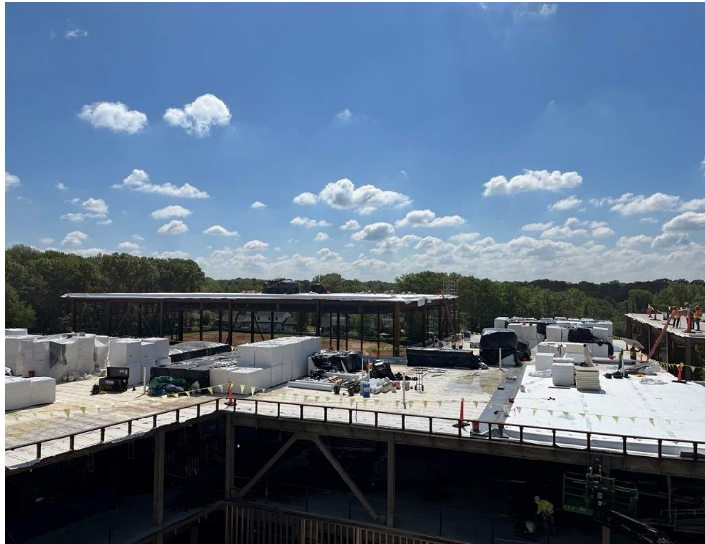
Roofing Area C
