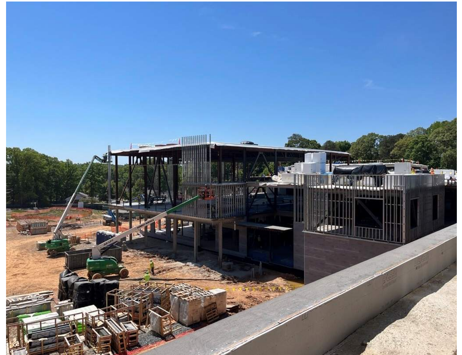
Area C Exterior Framing
