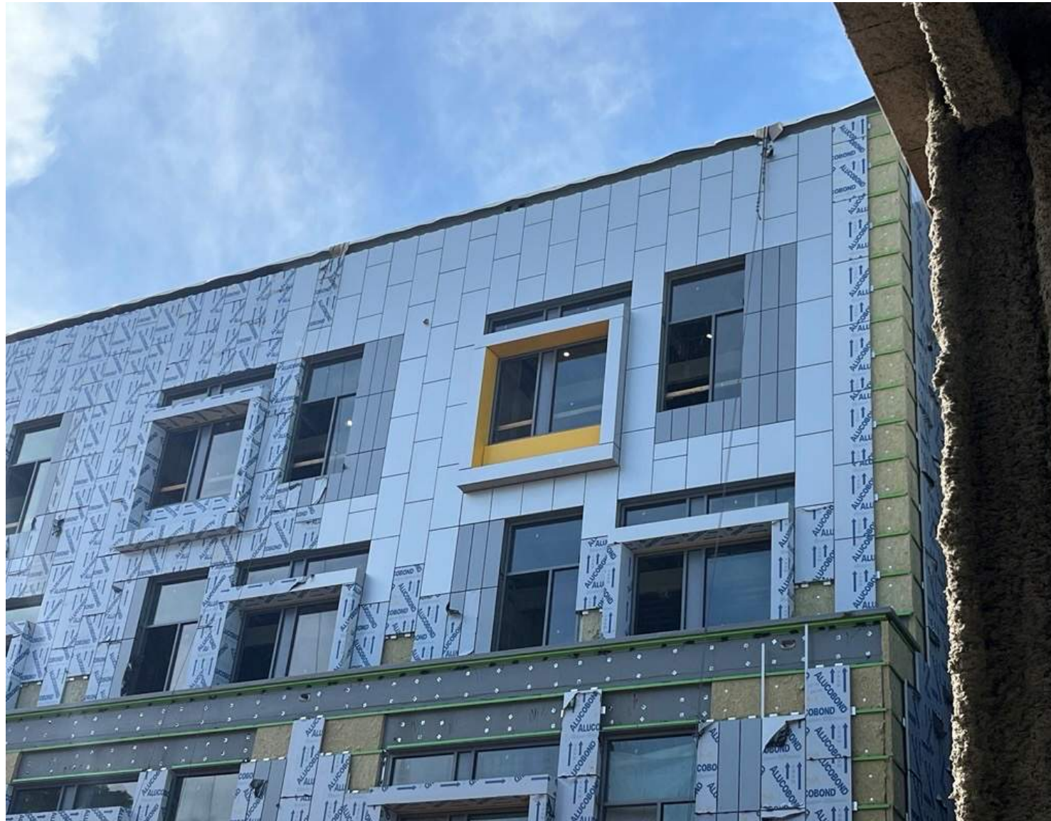
Area A South Elevation - Metal Panel and Windows
