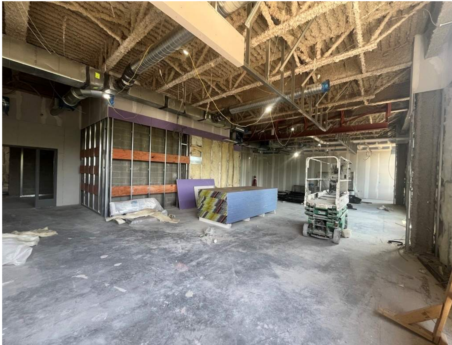
Classroom with Operable Partition
