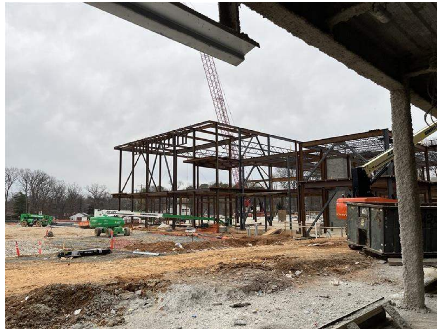
Area C Structural Steel
