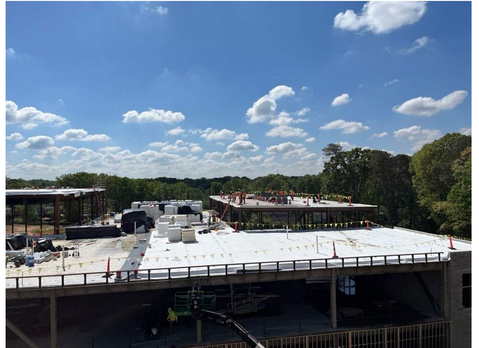
Roofing Area D
