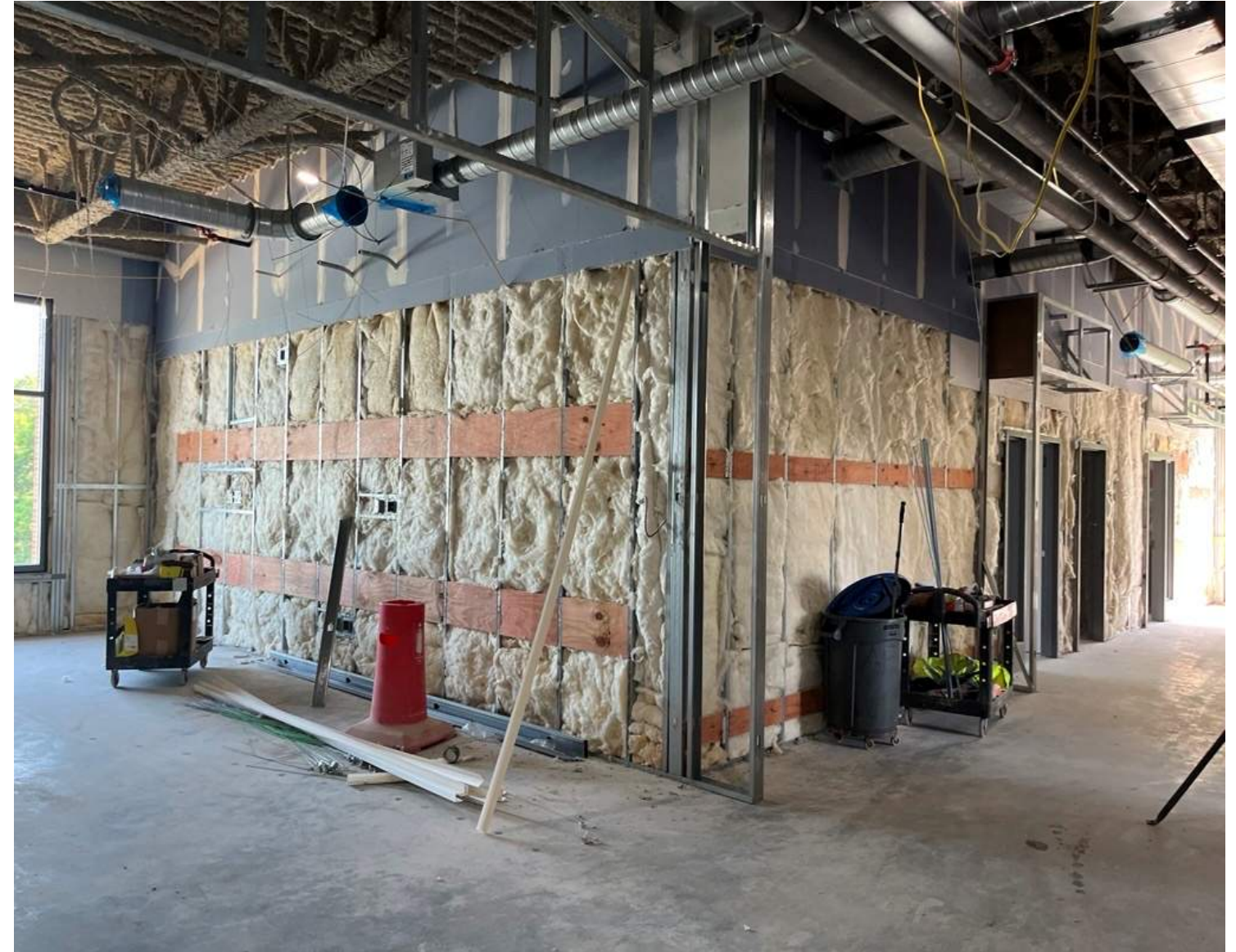
Drywall and Insulation in Area A
