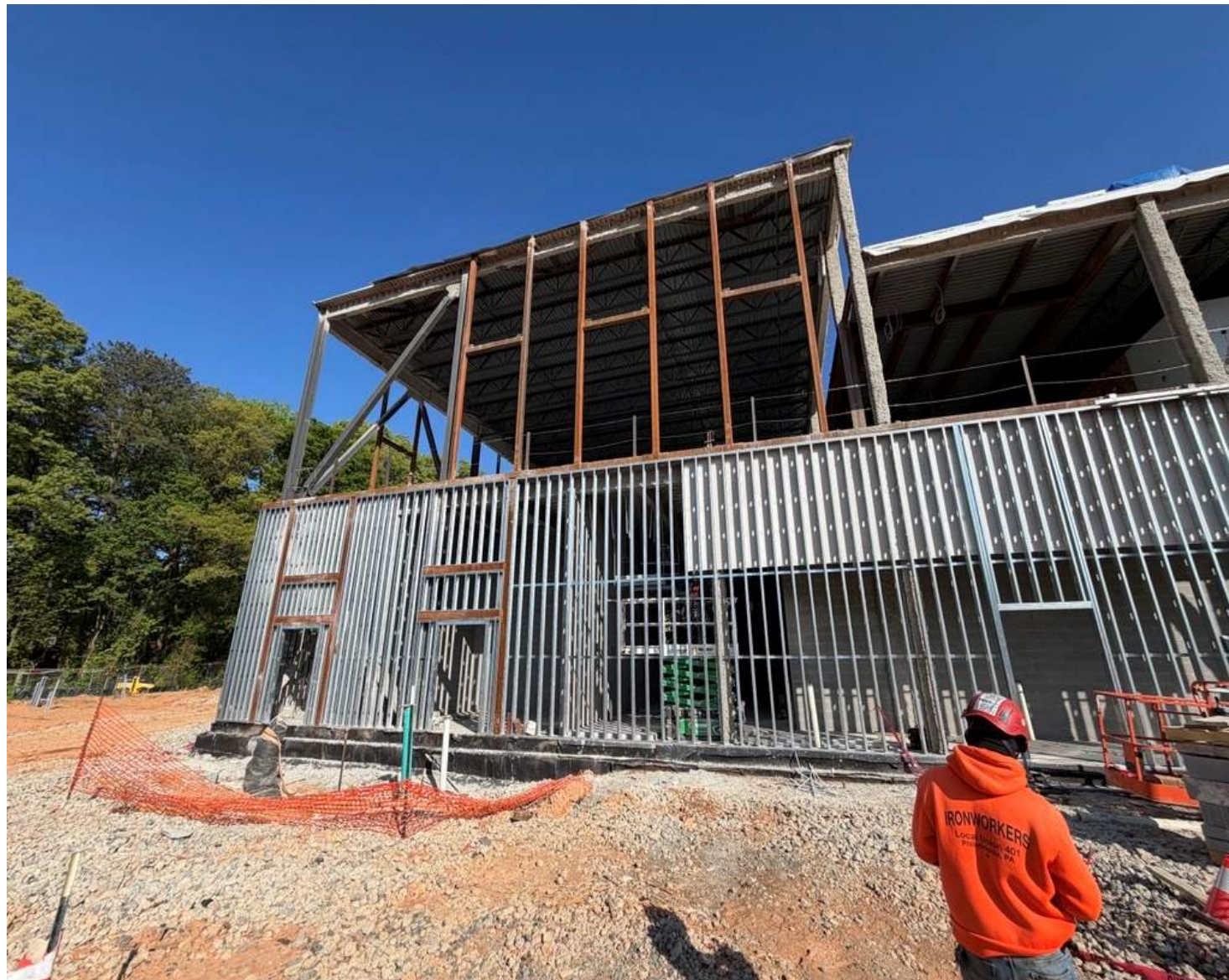
Area D Exterior Framing
