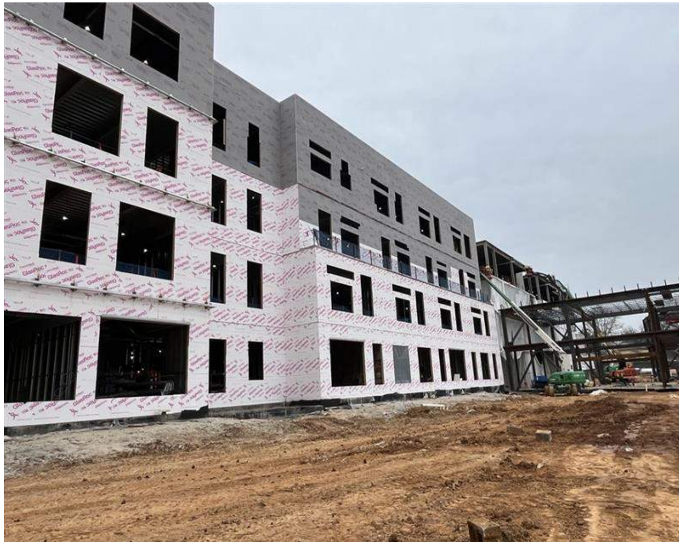
Area A South Exterior Framing
