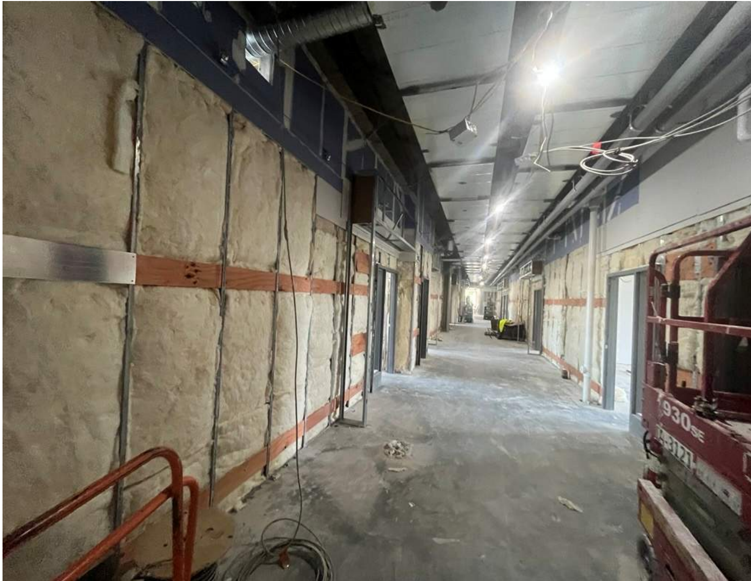
Drywall and Insulation in Area A
