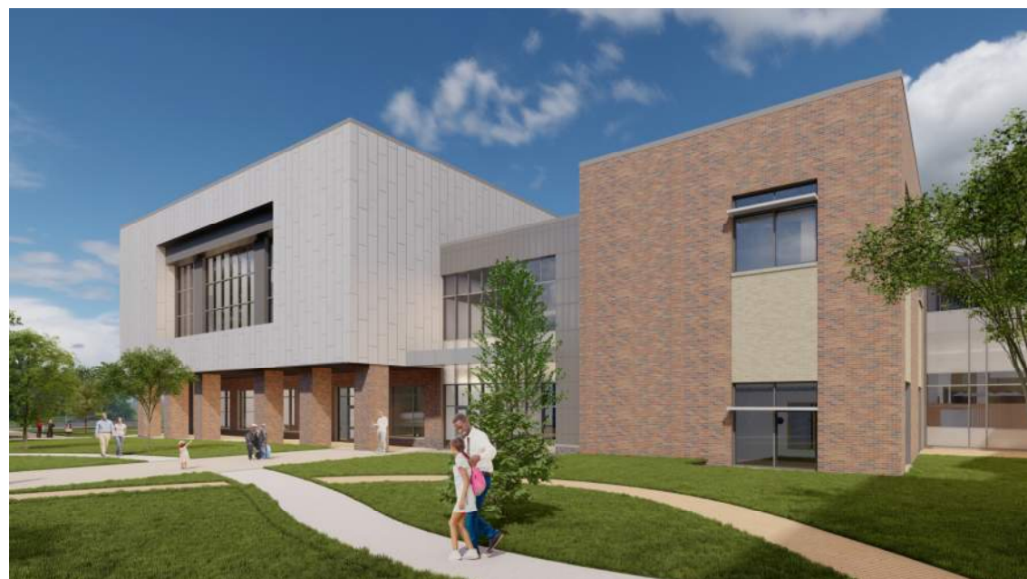
View of Community Entrance - Previous
