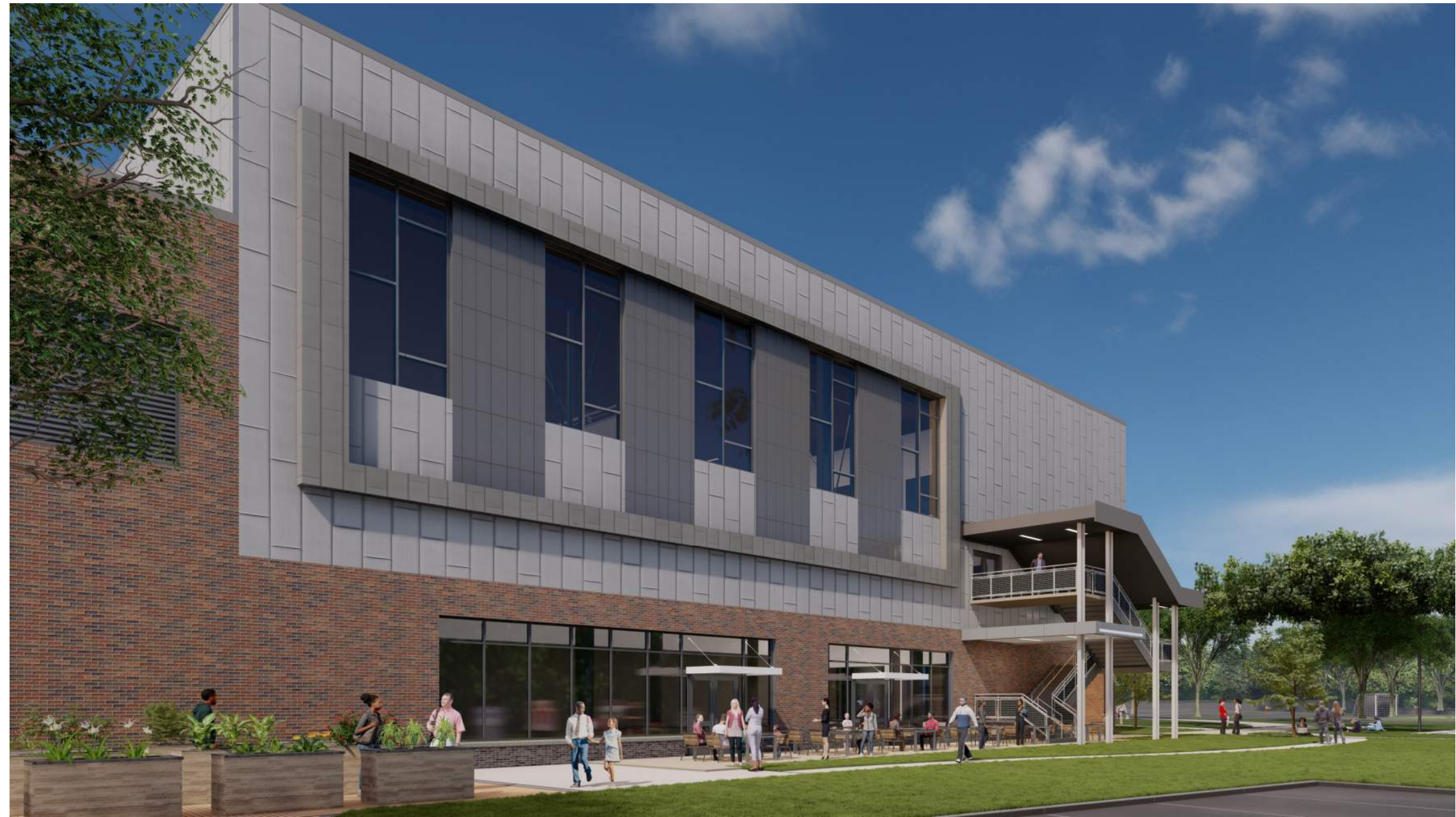
View of Gym Facade
